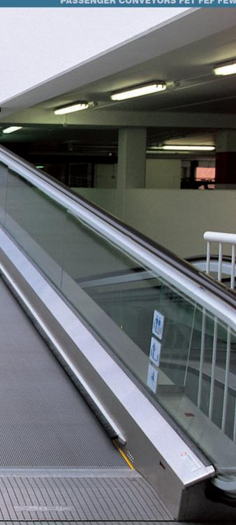
The **Moving Walkway** combines all the advantages of the escalator by adding the advantage of being able to carry the shopping or luggage trolleys. Also in this case the technological quality and sturdiness of the installation are combined to a lightweight design, completed by the colourless tempered glass balustrade (10 mm thick).
